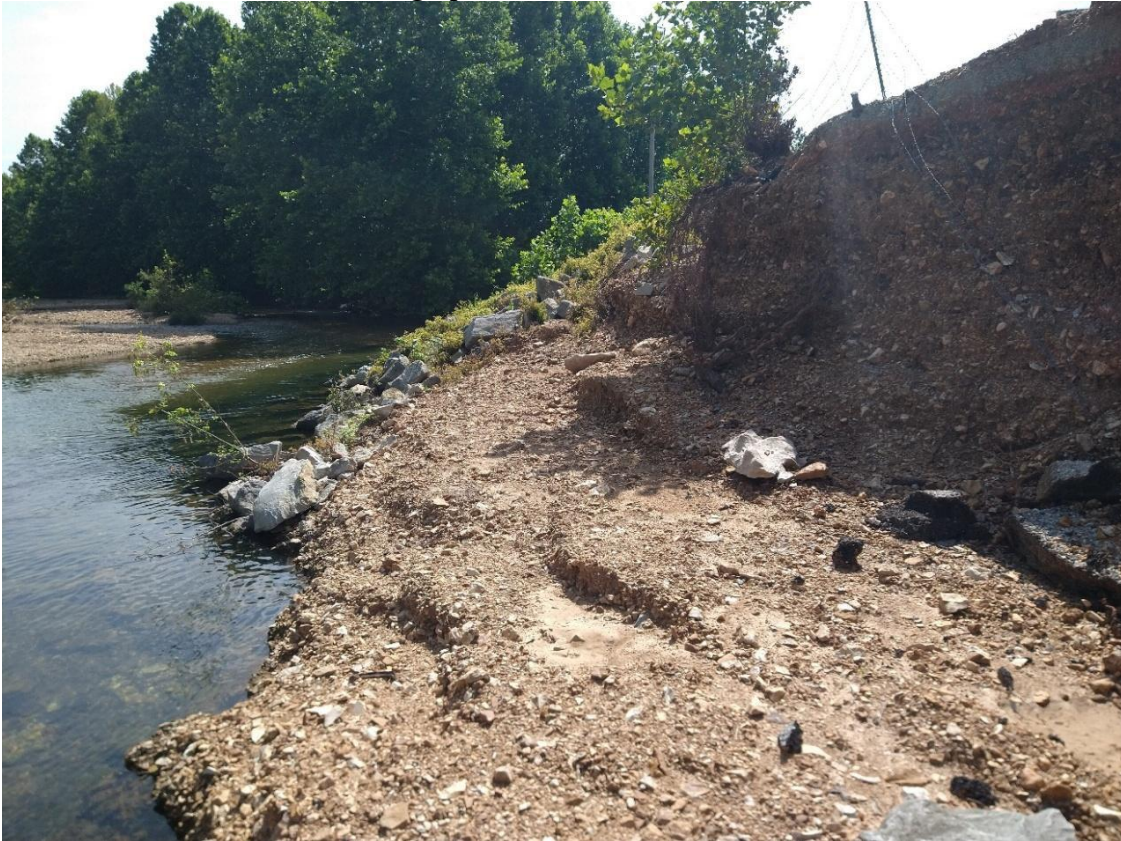
Picture #4 - Stream level looking south at the abutment wall with washed out approach material
