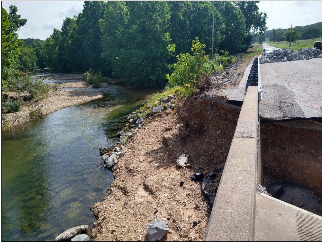
Picture #1 - North side of bridge looking upstream
