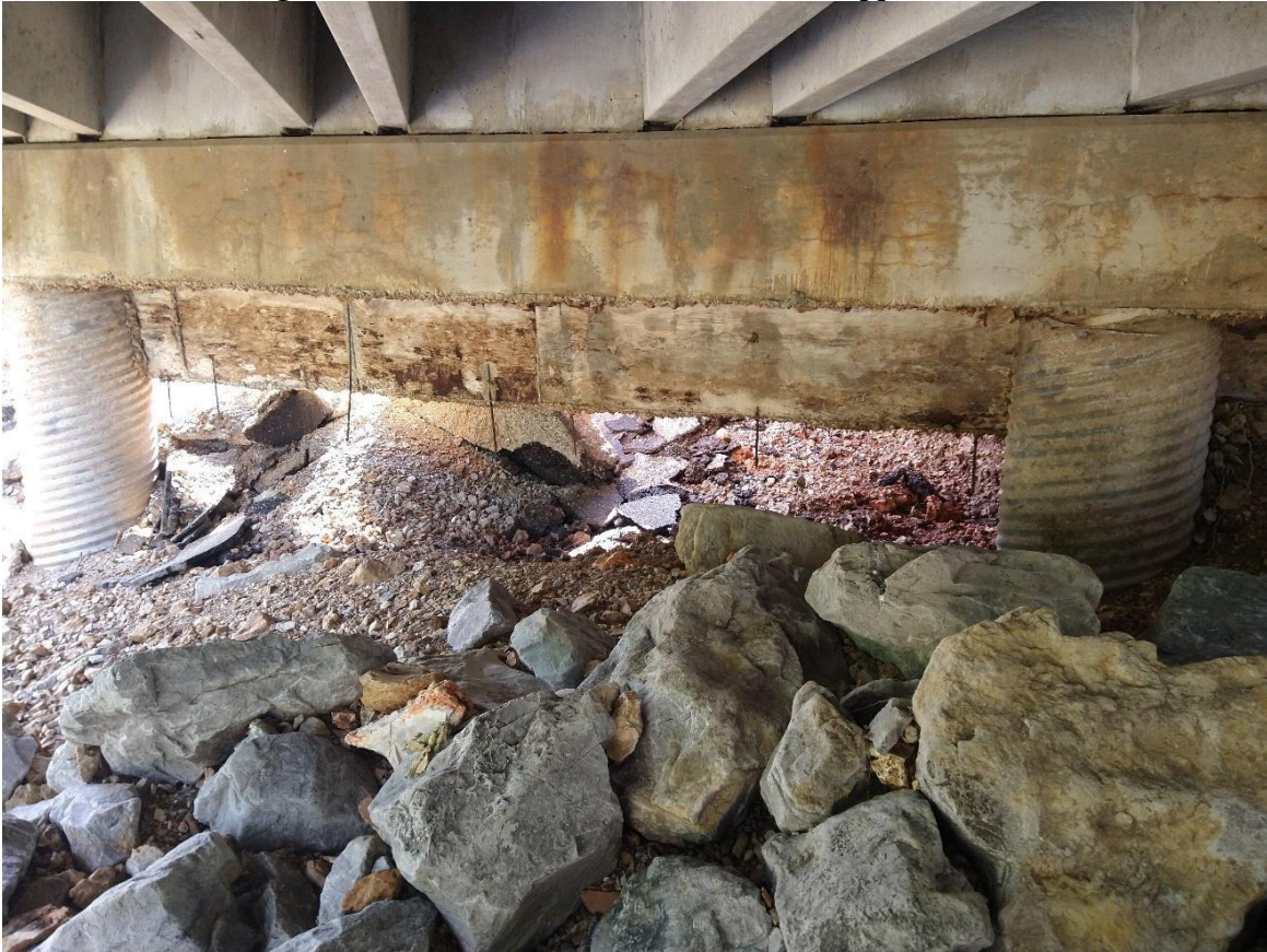
Picture #6 - South east end of bridge erosion around culvert
