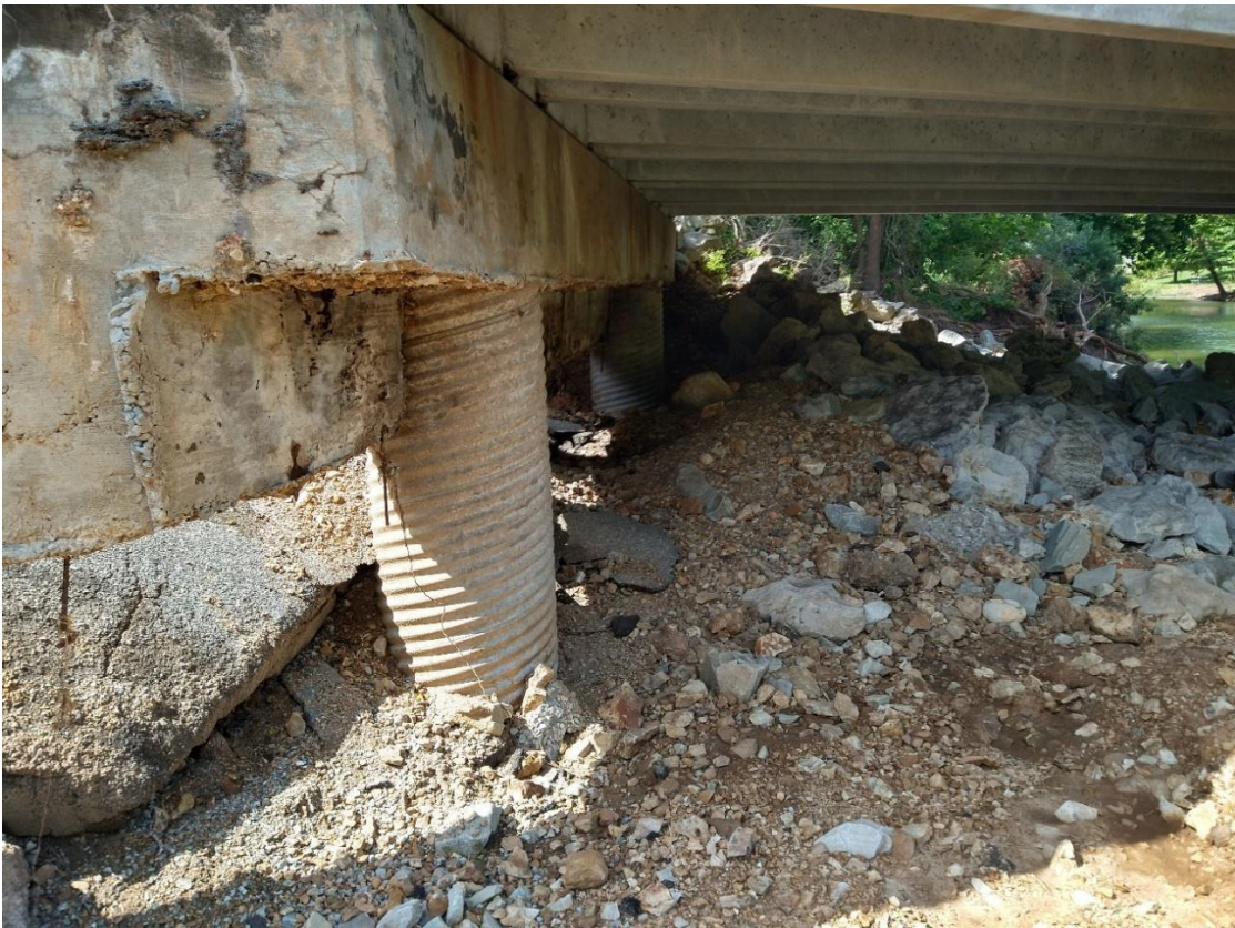
Picture #4 - Stream level looking south at the abutment wall with washed out approach material
