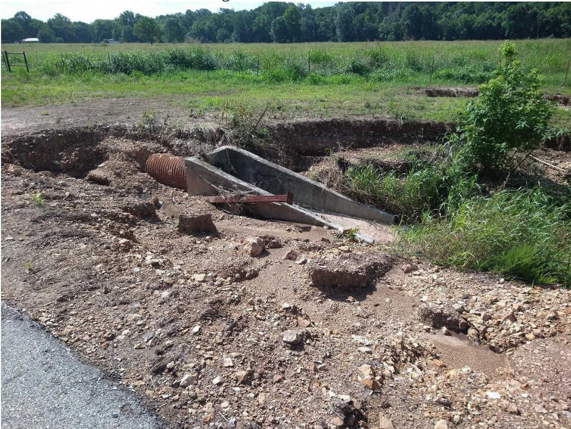
Picture #6 - South east end of bridge erosion around culvert
