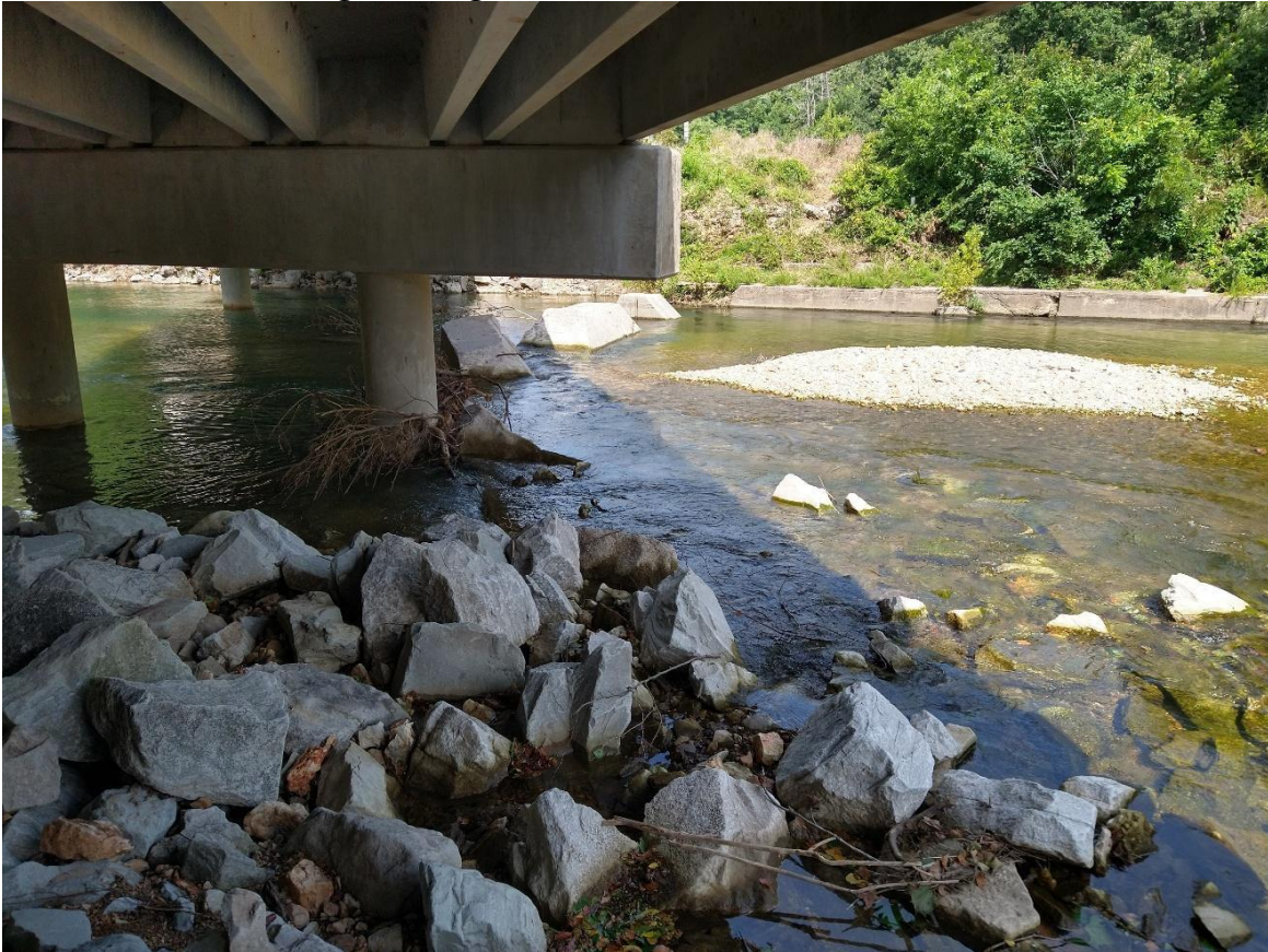
Picture #7 – Below bridge looking west
